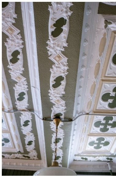
Figure 13: Detail of tin panel ceiling.
