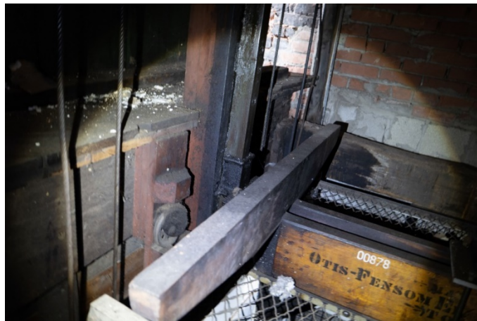
Figure 53: View of the elevator's wooden guide posts.
