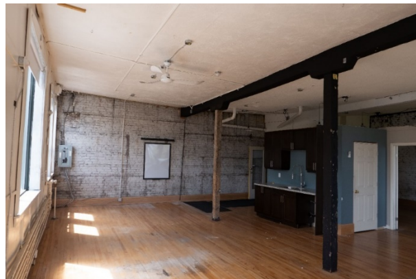
Figure 20: View of party wall and wooden posts at the second floor level.
