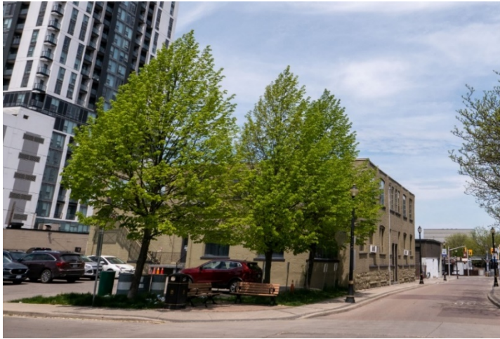
Figure 1. Looking north at the Radigan Building, set directly against Ferguson Avenue South.
