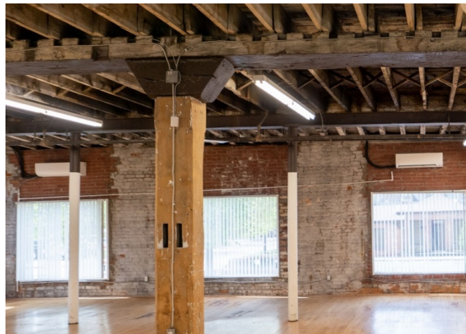
Figure 11: Detail of salvaged wood posts and beams, showing unused joist pockets and tenons.
