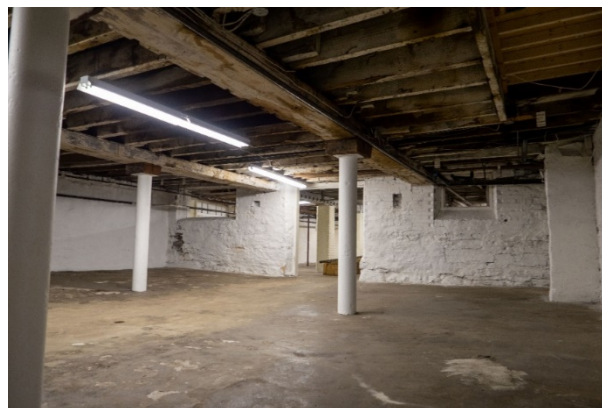
Figure 22: Looking southwest from the southeast quadrant, past the original rear foundation wall and window openings.
