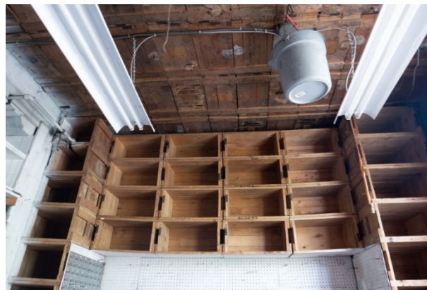
Figure 16: Re-used wooden boxes used as shelving and cladding in the rear workshop space.
