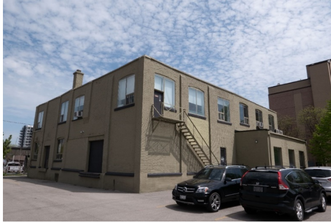
Figure 3: View to the south and west elevations of the Radigan Building.
