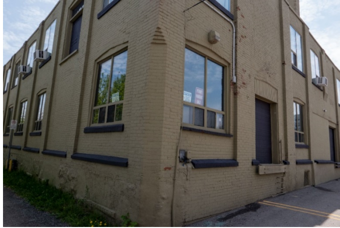
Figure 8: Decorative corbelling transitioning chamfered northwest corner.
