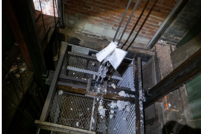
Figure 52: View of the elevator's open freight car.
