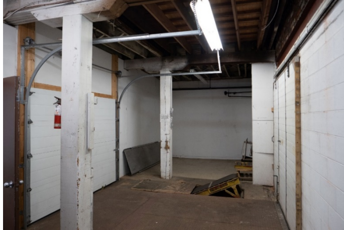
Figure 10: Smaller rooms at rear of 48 Ferguson use smaller posts and built-up beams.
