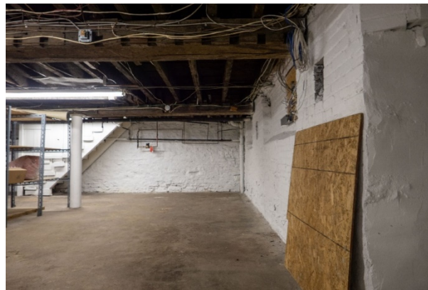
Figure 21: Looking south from the northeast quadrant of the basement at the party wall separating 46 and 48 Ferguson. The former rear foundation wall is at right, with previous window openings visible.
