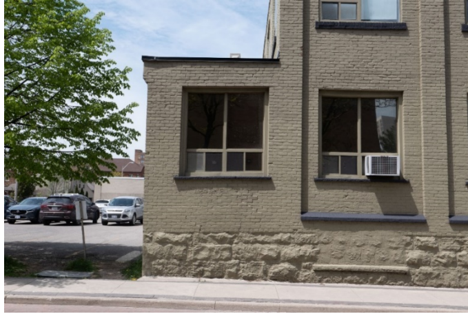
Figure 6: Non-original flat window openings seen on south end of the main elevation and south addition.
