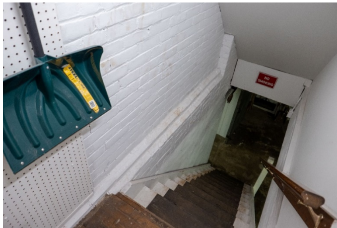
Figure 36: Former exterior wall shows water table and other brick details.
