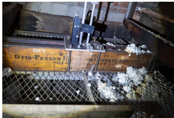
Figure 19: Otis-Fensom top beam of the elevator car.
