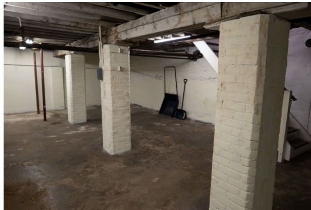
Figure 24: Brick posts supporting built-up beams in the southwest quadrant.
