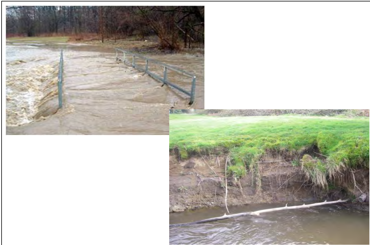
Figure 5.3: Flooding and Erosion Impacts
